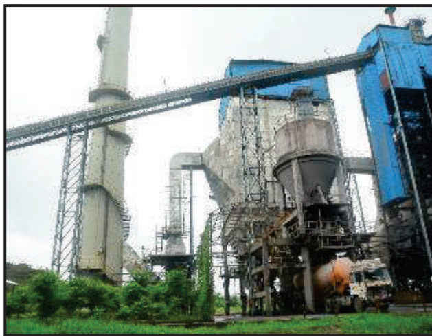
Photo Showing Line-1 Cooler ESP
