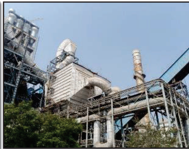
Photo Showing Line-2 Cooler ESP
