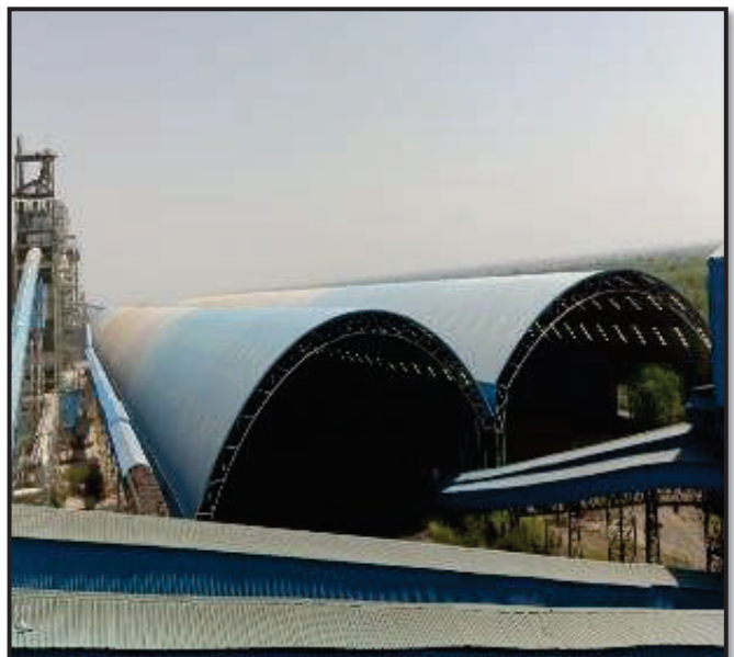
Photo Showing fly ash Silo
