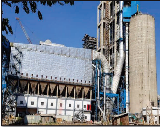
Photo Showing Raw Mill + Kiln Line- 3 RABH
