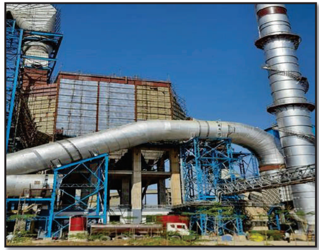
Photo Showing Line-3 Cooler ESP
