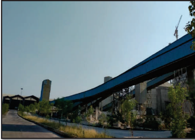
Photo Showing Covered conveyor belt
