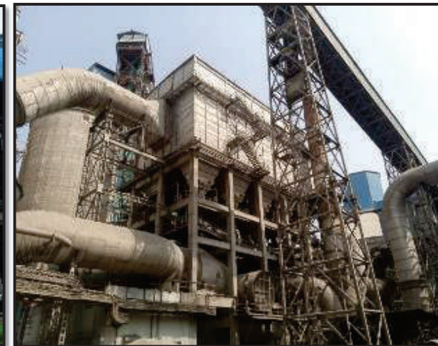
Photo Showing Line-2 Cooler ESP
