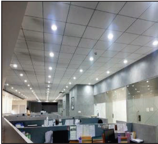
Photo Showing LED light fixtures at Office
