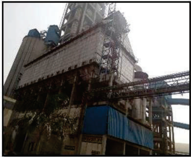
Photo Showing Line-2 RABH
